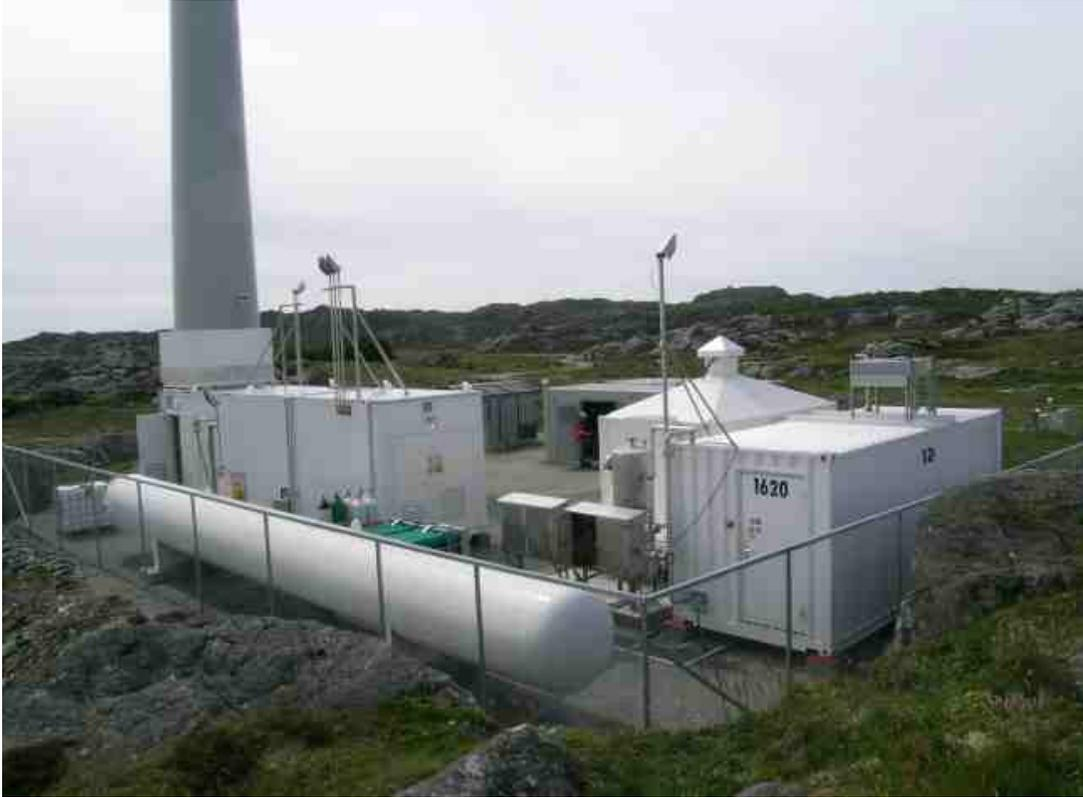
*Figure 2 Photograph of the wind-hydrogen power plant at Utsira. Below the tower: the electrolyser and compressor container. In the front: the H<sub>2</sub>-storage tank. To the right: the fuel cell and H<sub>2</sub>-ICE container. In the background: the grid stabilizing equipment.*
