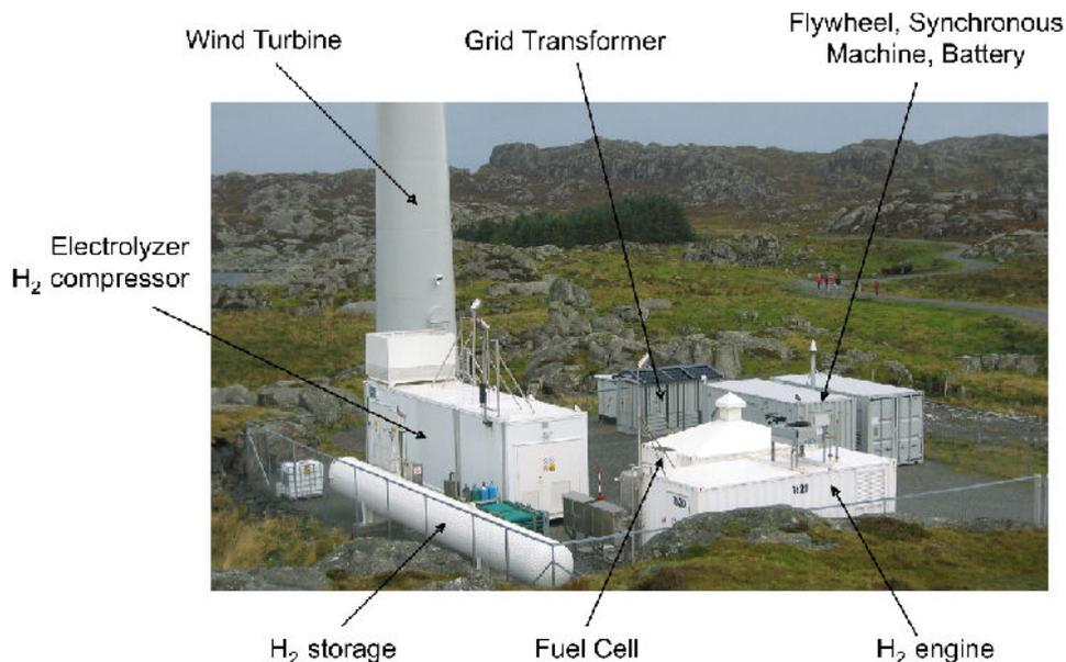
Figure 1: Wind/hydrogen energy system at Utsira, Norway (Photo: Ulleberg, 2005)
