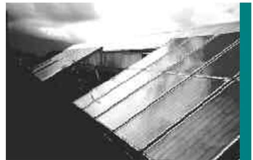
Solar heating panels used in the greenhouses at El Golfo. The 100% renewables strategy not only concerns electricity production. At the same time, El Hierro has started to develop an ambitious programme to harness solar-thermal energy for producing hot water, and, in the near future, for cooling, and for implementing stand-alone photovoltaic systems in isolated ones and others that are connected to the grid.
