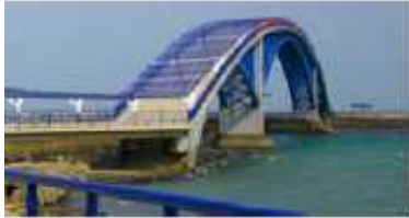
Bridge with Photovoltaics
