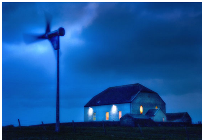
Figure 5 – Westray Parish Kirk and 6kW wind turbine
